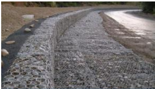
River bank protection
