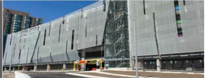
PARKING GARAGE CLADDING
